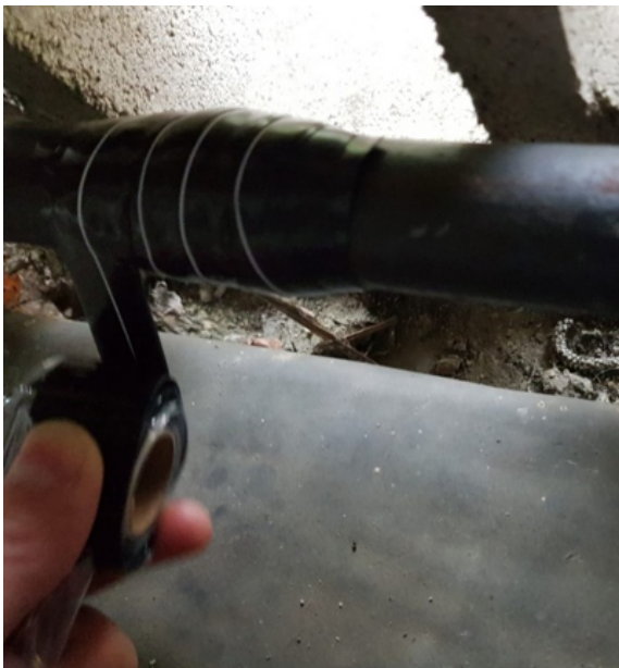
The tape was then pulled under the pipe and up through the 30mm gap between the pipe and the back wall. Despite not being stretched to its limit, Wrap & Seal still amalgamated to form a solid rubber band
