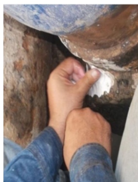
Superfast Aqua PW sealed a tee-joint by filling all gaps in the connection with a rock-hard material
