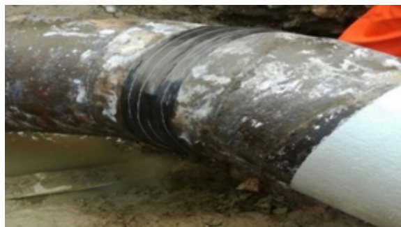
Wrap & Seal was used to repair a leak on an elbow bend which could not be isolated
