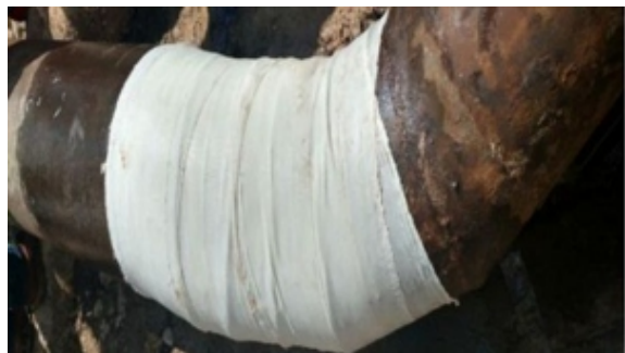
SylWrap HD reinforced the Wrap & Seal repair
