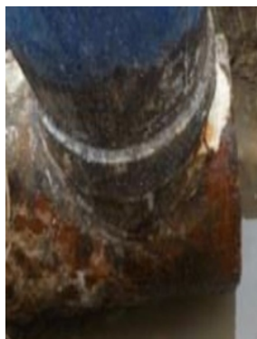
Superfast Aqua PW sealed a tee-joint by filling all gaps in the connection with a rock-hard material
