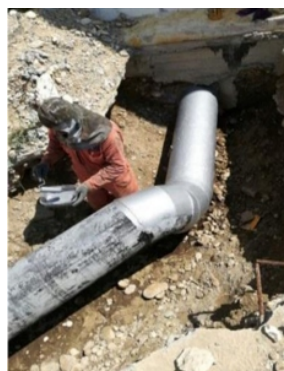
Liquid Metal created a new outer surface protecting and strengthening weakened areas of the pipe
