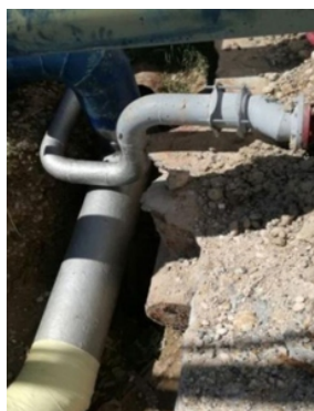
Liquid Metal created a new outer surface protecting and strengthening weakened areas of the pipe
